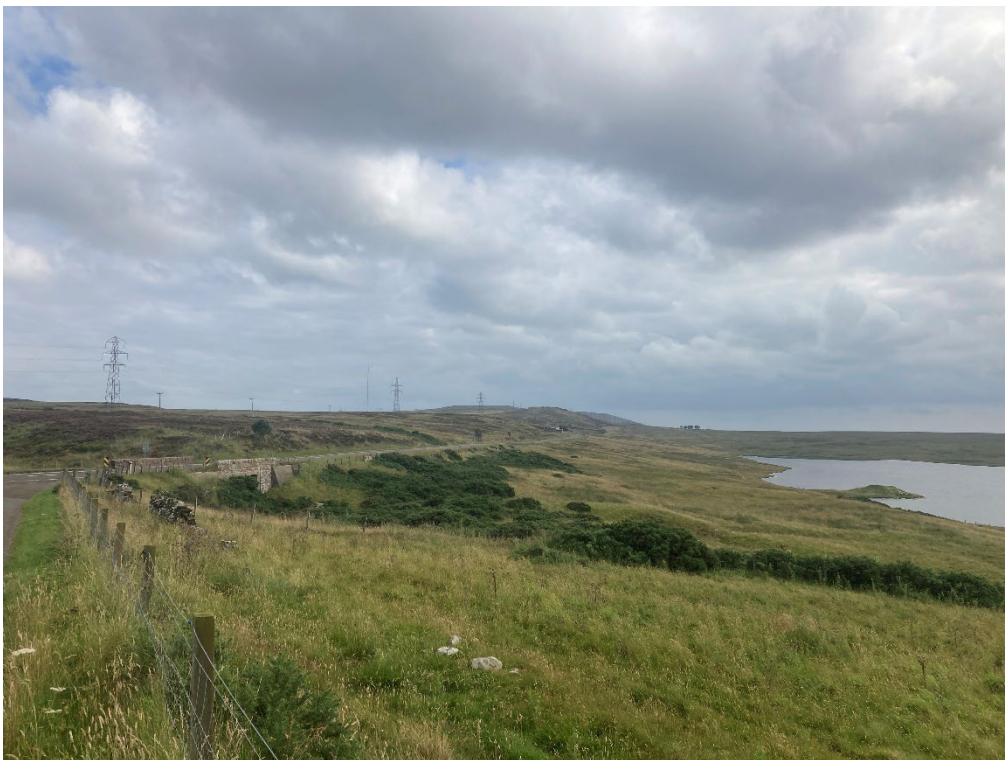
Photograph 5.2-21: View south along the A9, with Loch Rangag and Greysteil Castle Broch (SM555) right of image. The existing OHL as well as other infrastructure including the telecommunications mast on Ben-a-Chielt are visible along the ridgeline left of image.
